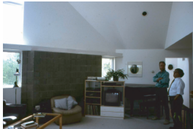
Living Room Trombe Wall
